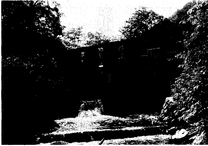
Photo 1. Gauging weir of SHOZAWA Basin.
